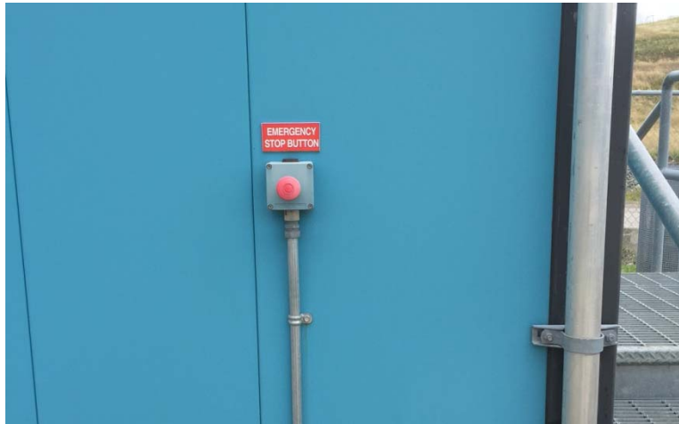
FIGURE 4 - FLARE STATION EMERGENCY STOP BUTTON
