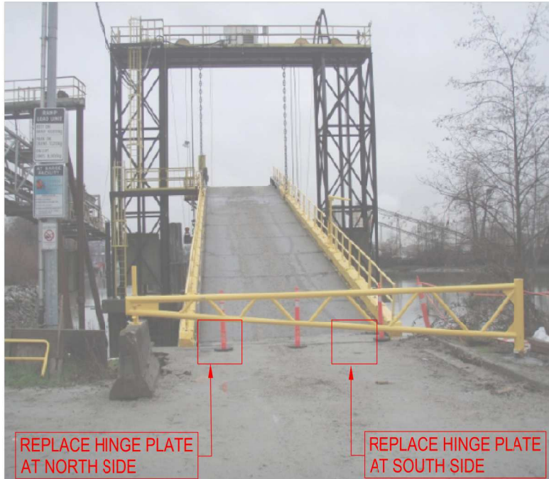
PHOTO - BARGE RAMP REPAIR LOCATIONS
