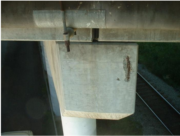
Fig 5. Corrosion of reinforcement causing spalling of the concrete at the top of the pier
