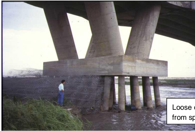
Fig 3 – Extensive scouring at a bridge pier
