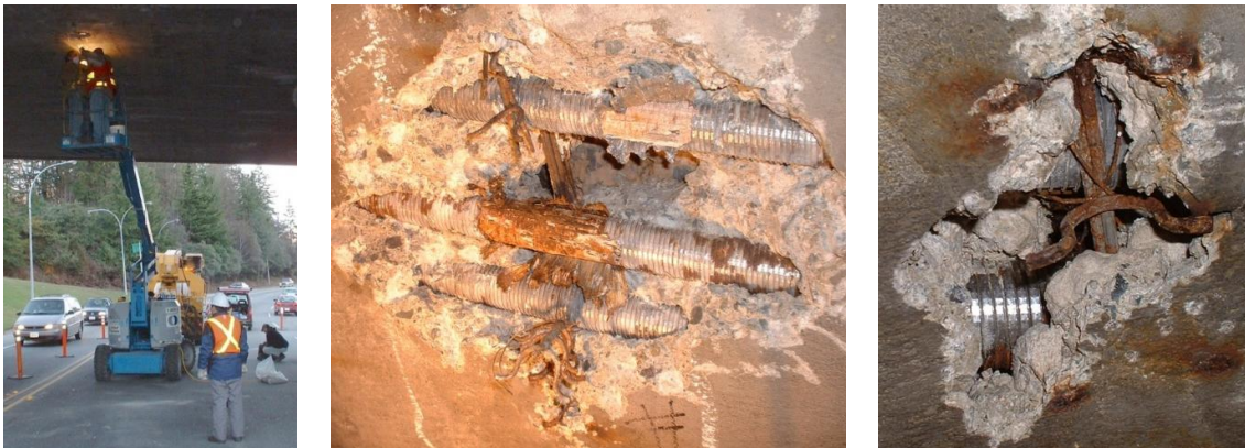
Fig 7. Hammer sounding of underside of deck revealed a critical defect
