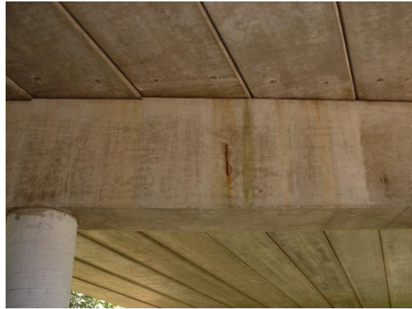
Fig 6. Note Algae on sides of top of pier from water leaking through defective expansion joint
