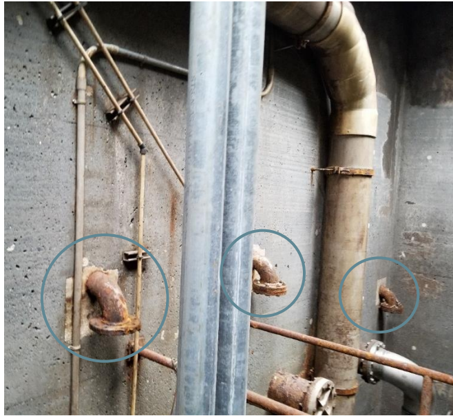
Figure 8: 100 mm dia. wet well flush pipes
