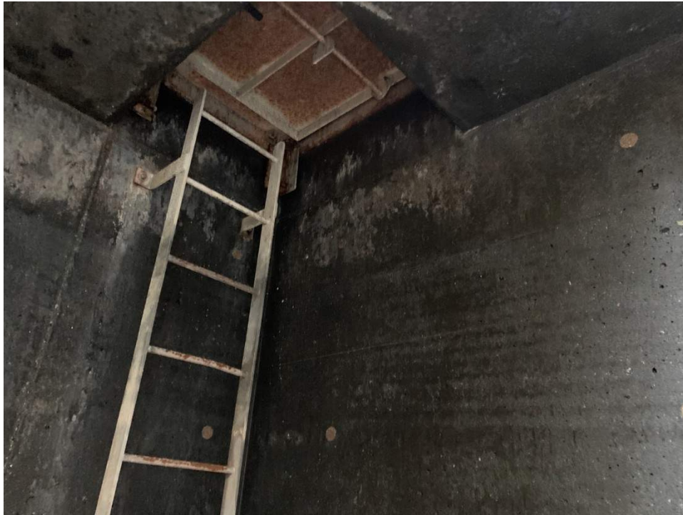
Photo 11: South-west ladder and access hatch. Appears to be some leakage around hatch.
