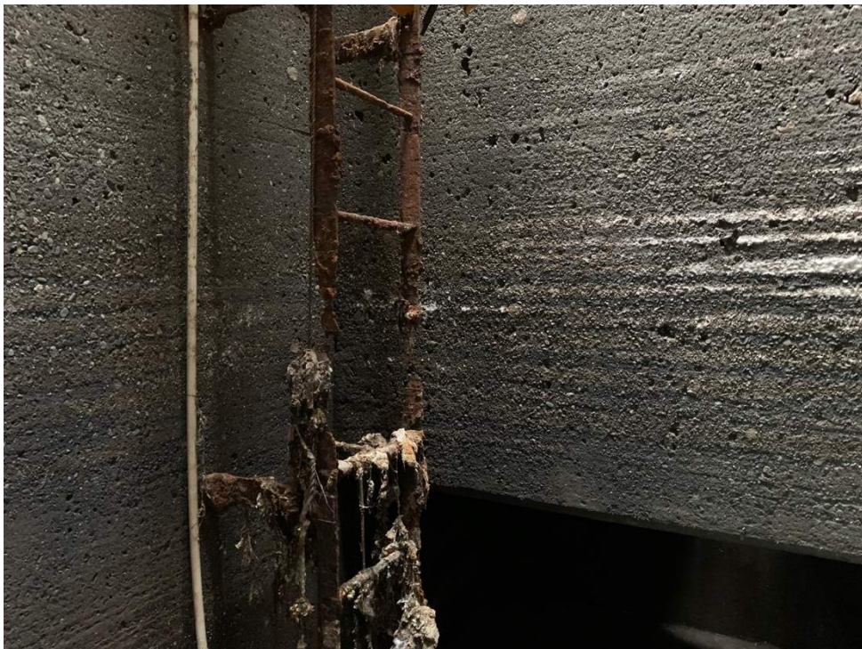
Photo 12: Lower ladder, very poor condition, complete section loss through side rail
