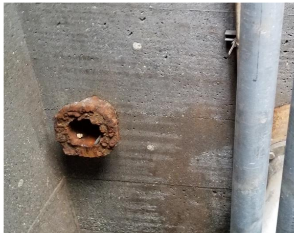
Figure 7: 200 mm dia. blowdown connection
