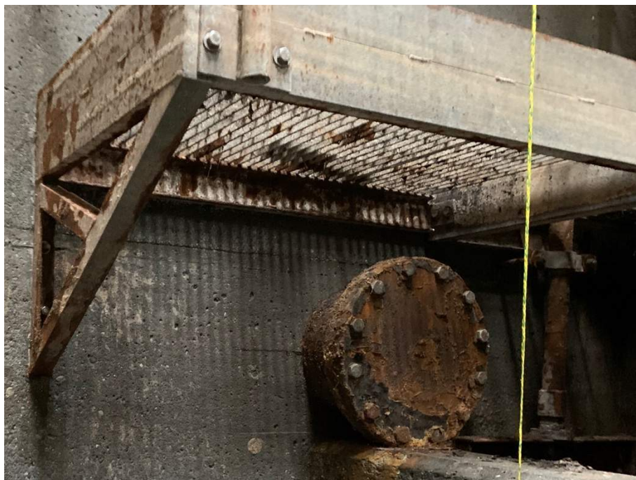
Photo 8: Intermediate platform, supporting steel in fair condition. Anchors to concrete appear stainless steel and with no visible corrosion.
