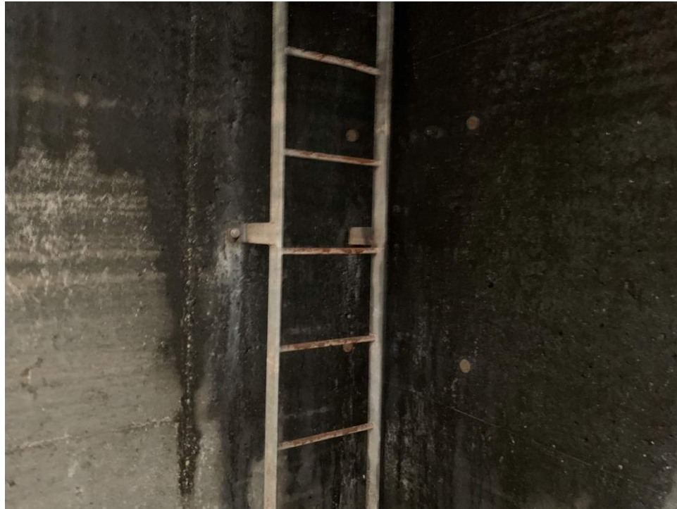
Photo 9: Upper ladder, good to fair condition, limited surface corrosion only.
