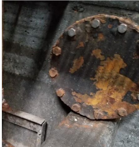
Figure 6: Overflow piping (blind flange installed)
