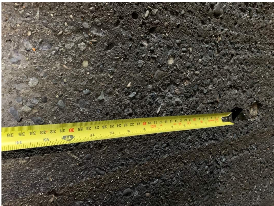
Photo 6: Maximum observed erosion of concrete surface, lower walls of wet well
