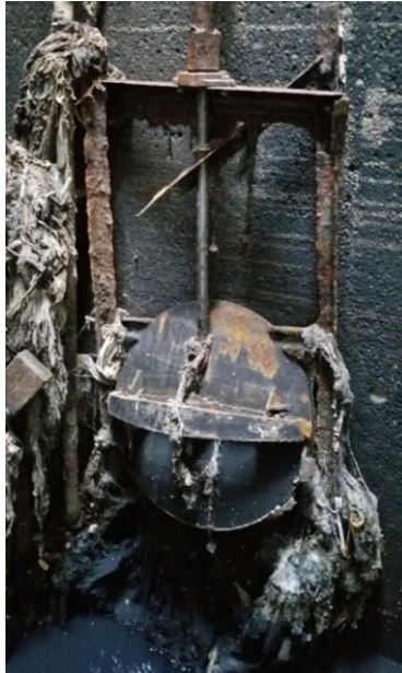
Figure 5: SG-4 Wet well dividing wall gate
