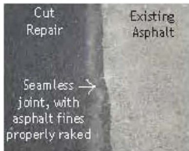
ACCEPTABLE SEALED EDGE OF CUT REPAIR*
