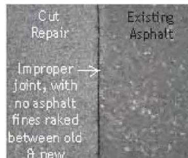
UNACCEPTABLE SEALED EDGE OF CUT REPAIR*
