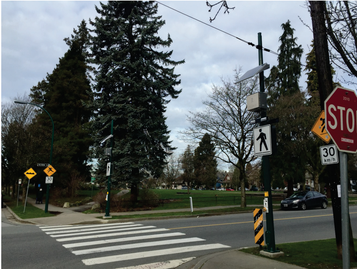
Figure 10-12: Rectangular Rapid Flash Beacons
