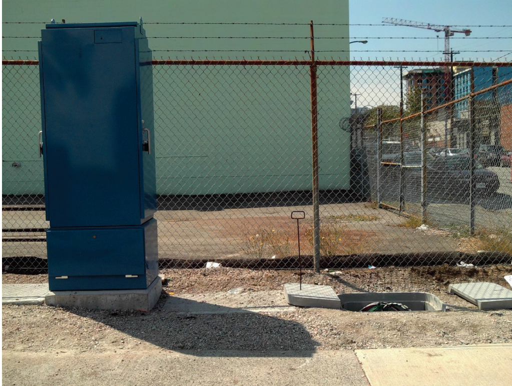
Figure 10-18: Type 332 Controller Cabinet with Battery Box
