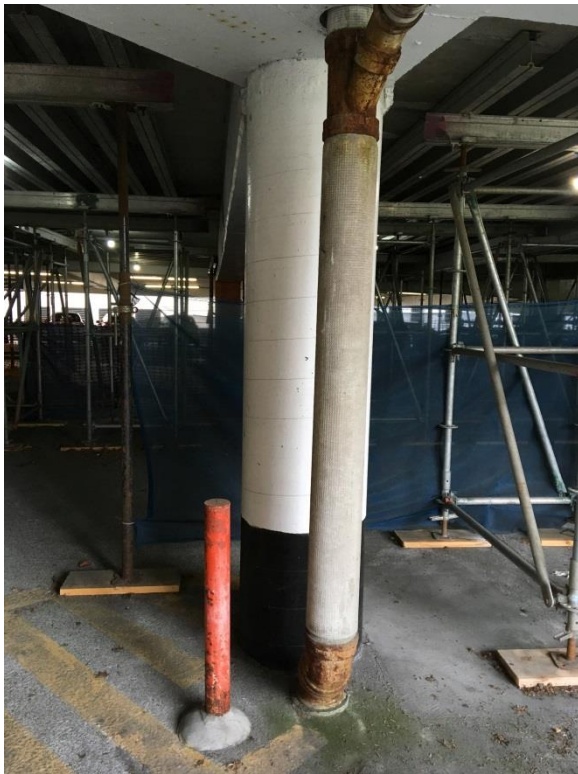
Photo 7: Presumed-Asbestos Cement Pipe
