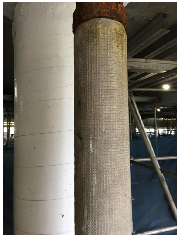
Photo 8: Presumed-Asbestos Cement Pipe
