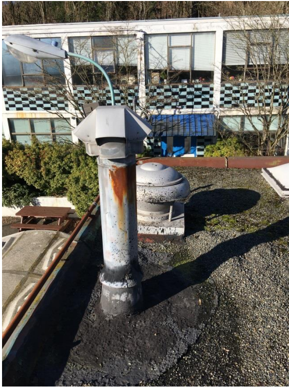
Photo8: East Roof(SE) - Black Tar on Vent Collar [7311-A08]
