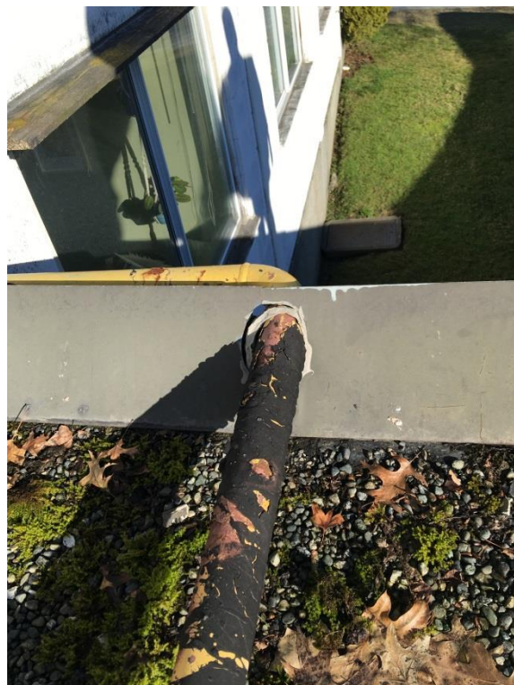
Photo11: Middle Roof - Grey Caulking Around Gas Pipe [7311-A13]
