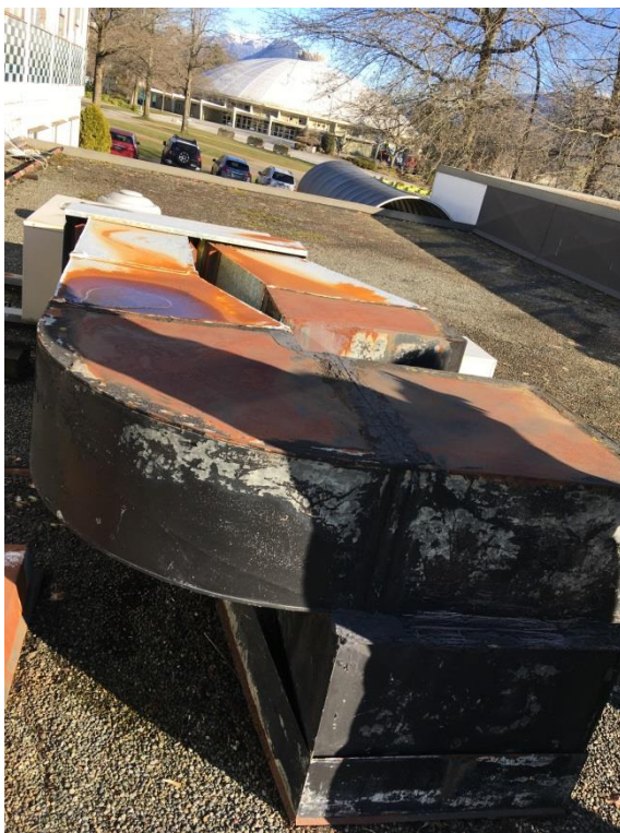
Photo10: Middle Roof - Black Tar on HVAC Duct [7311-A11]
