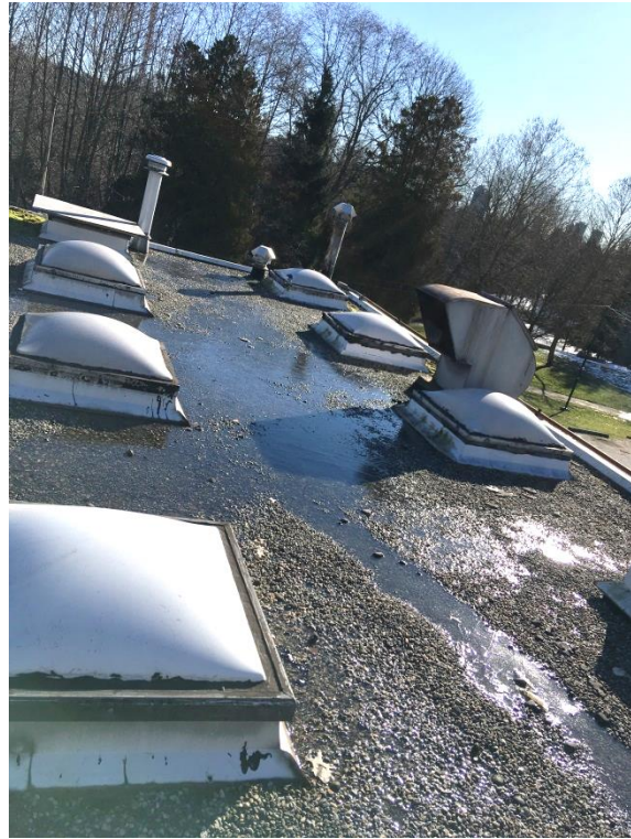
Photo9: East Roof (SE) - Black Tar on Skylights [7311-A09]
