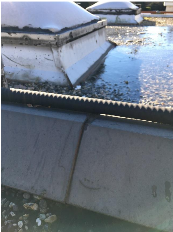
Photo6: East Roof (N/S) - Grey Mastic on Metal Flashing [7311-A06]
