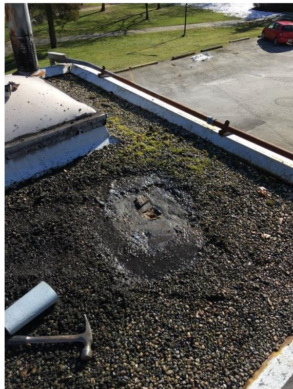
Photo3: East Roof(SE) - East End Roof Test Cut [7311-A03]
