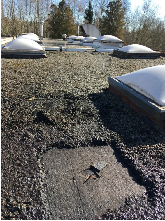
Photo4: East Roof (SW) - West End Roof Test Cut [7311-A04]
