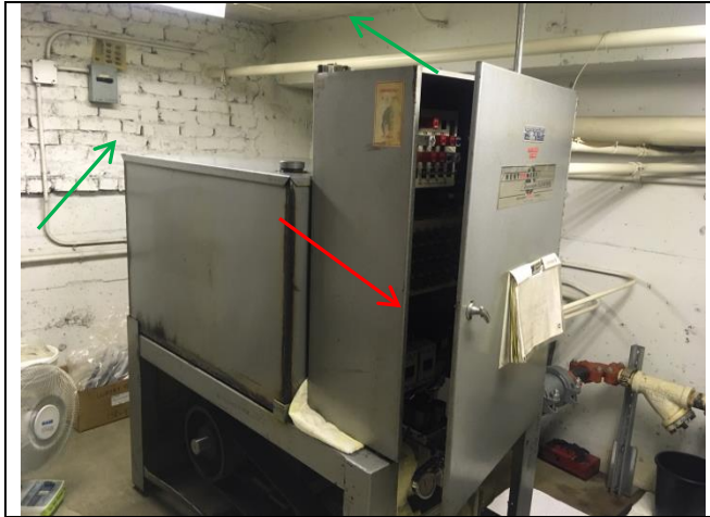
Photo 1: Grey paint on Metal Elevator Machine Equipment is lead containing. Paint on walls and ceiling throughout is not lead containing. Brick mortar is also non-asbestos.
