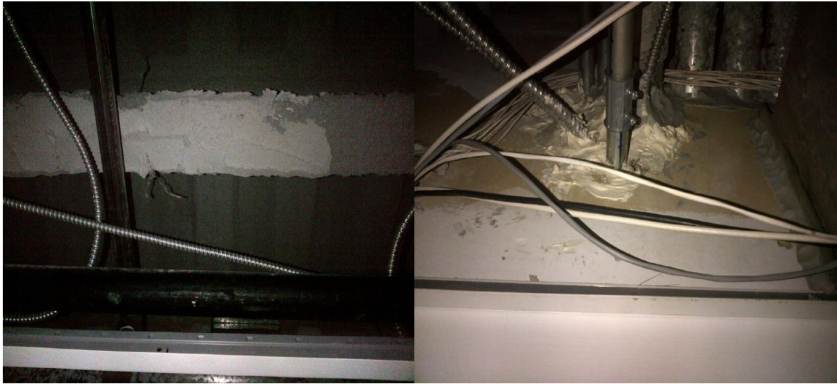
555 – Floor 2 (Above ceiling space)
