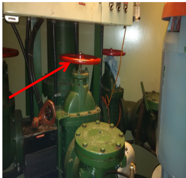
Photo 3: Red Paint on Valve Handles and Pump Housings - Lead Based Paint
