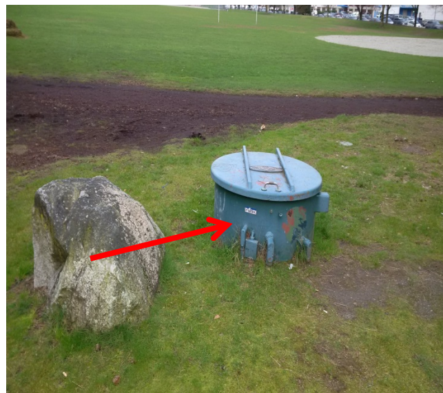
Photo 1: Multi color paint layer on Exterior Entrance - Lead Based Containing.
