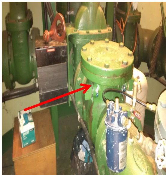
Photo 2: Mechanical System - Lead Based Containing and Presumed Asbestos Containing Gasket.
