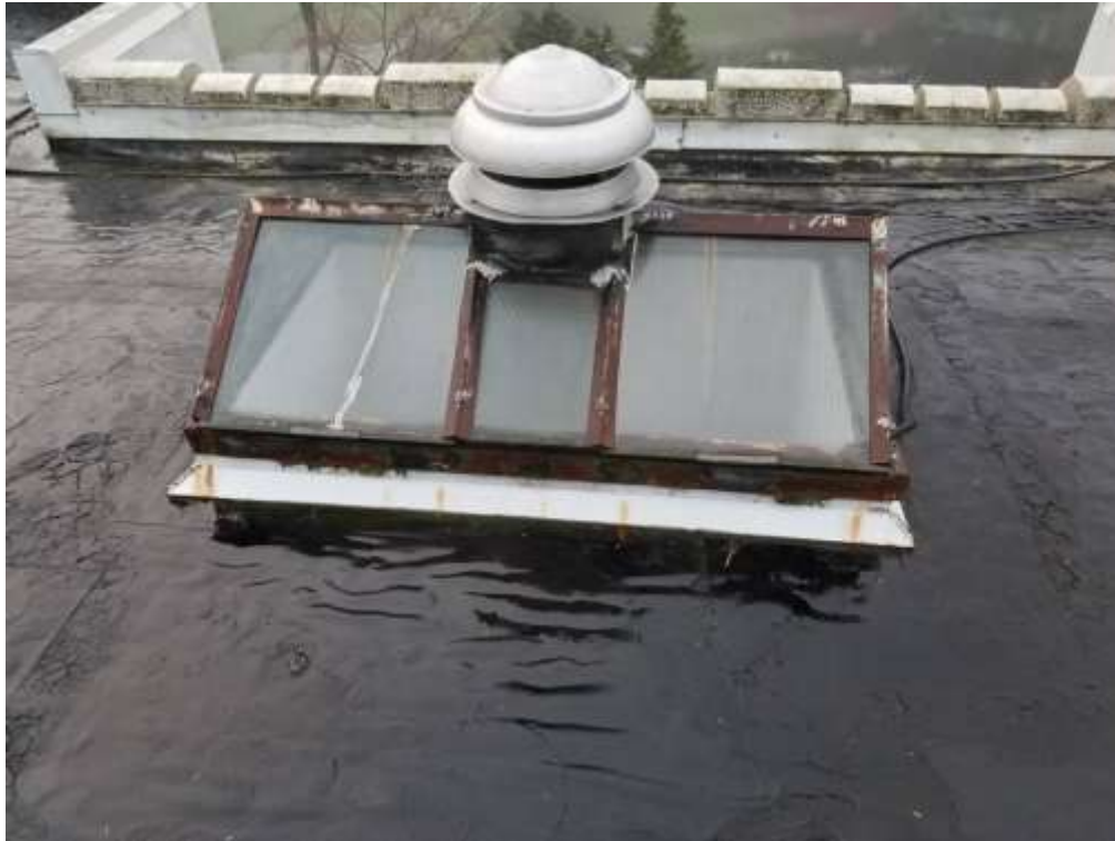
Photo # 1 – Asbestos-containing mastic on the skylight – upper roof, south section
