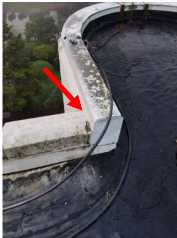
Photo # 2 – Asbestos-containing caulking between the metal flashing and exterior wall
