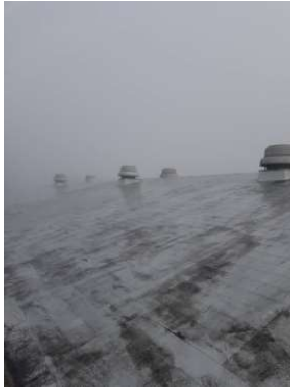
Photo # 5 – Upper exhaust flashings that were inaccessible during our investigation, all caulking are assumed to be asbestos-containing
