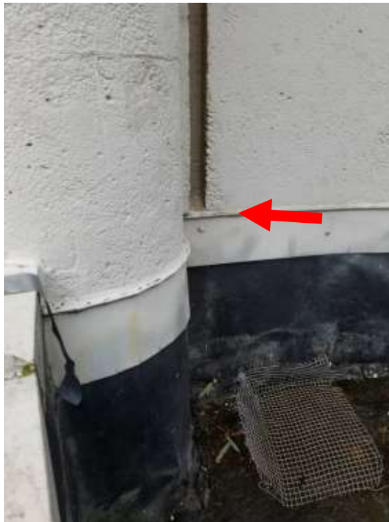
Photo # 4 – Asbestos-containing caulking between the metal flashing and exterior wall
