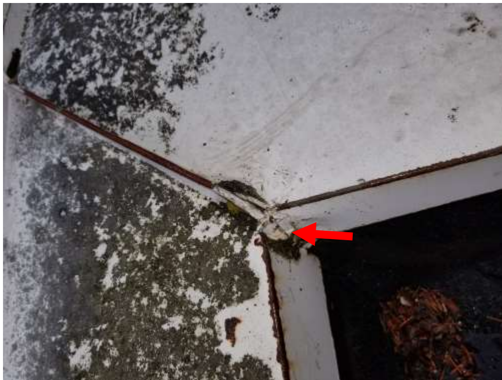
Photo # 6 – Asbestos-containing caulking on the perimeter metal cap flashing
