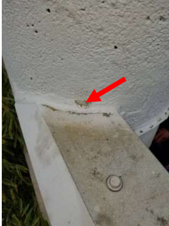
Photo # 3 – Asbestos-containing caulking between the metal flashing and exterior wall
