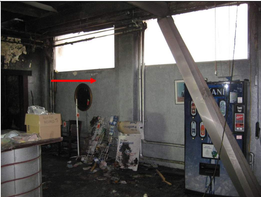
Photo 14 | Date: February 2014 | Location: Zone 2 - North wall of the reception/front desk area Description: Textured Cement Screed/Stucco, Sample# B00557-14 ASBESTOS-CONTAINING
