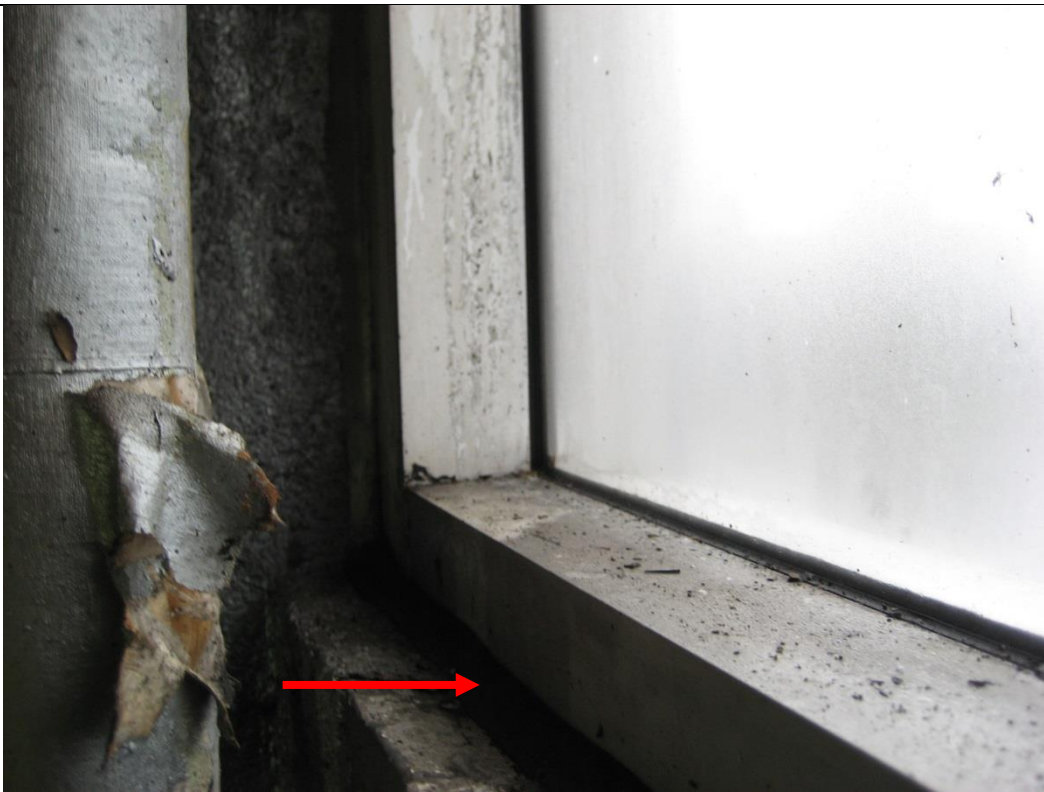
Photo 13 | Date: February 2014 | Location: Zone 2 - North wall, window frames Description: Mastic, Sample# B00557-13
