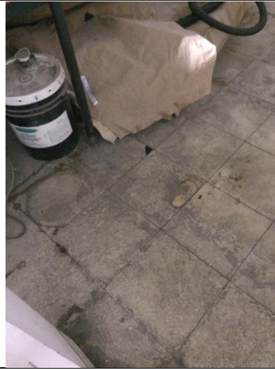
Photo 2: Non-asbestos containing 12" x 12" beige floor tiles with non-asbestos underlying mastic
