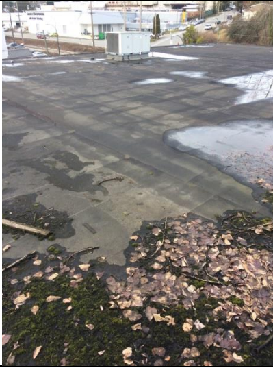
Photo 1: Non-asbestos containing roofing material
