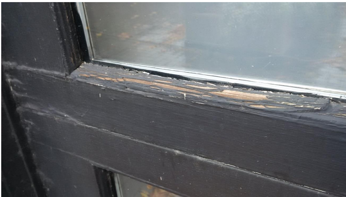
Photo1: Lead Based Black Paint On Wooden Garage Doors (South East Side of Building).
