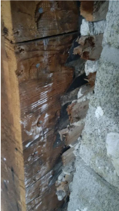
Photo4: NON-Asbestos Black Insulation Paper Behind Exterior Walls
