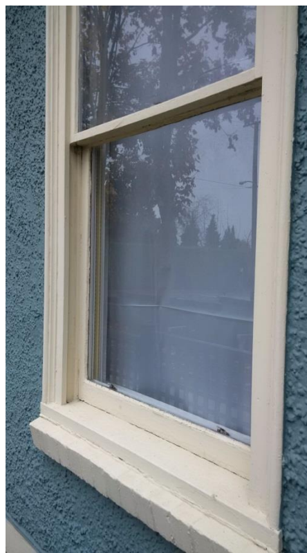
Photo3: Lead-Containing Beige Paint on Wood Trim
